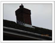
There is one brick built chimney stack. These show general weathering but condition was consistent with age. Condition rating 1
