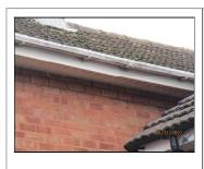
The timber soffit and fascia boards have been clad with plastic. Plastic cladding shows signs of general weathering but were considered to be in serviceable order. Condition rating 1. The original timber joinery is now hidden from inspection. It is not possible to comment on the condition of timber joinery hidden by plastic cladding.
