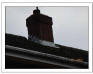
Rainwater goods are of plastic construction. Evidence of leaks and congestion/overflow were noted to gutters/downpipes. Rainwater goods show some general weathering and should be subject to routine overhaul to include removing debris, re-sealing joints and re-alignment as necessary. Condition rating 2.
