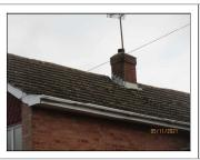
The main sloping roof is covered with tiles over a secondary waterproof barrier. There is evidence of general weathering, however the condition was considered to be consistent with age. Condition rating 1.
